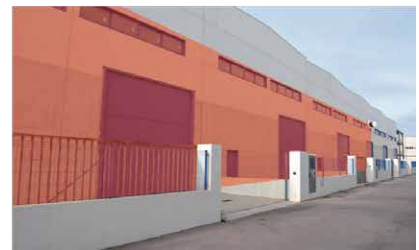
Wall protection (outdoor) at Warehouse
