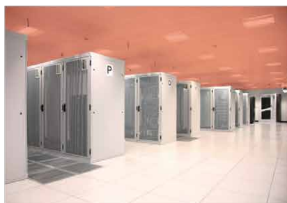
Ceiling protection at Data center
