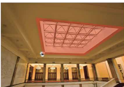
Skylight protection at Public facility / Warehouse
